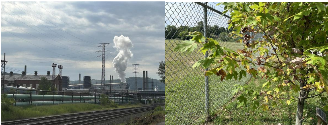
Fig. 1. (Left) Quenching of a coke battery at the Clairton Coke Works on July 20, 2024. "Wet" quenching dumps water on coal that has been heated to 1800 F for nearly a day, releasing hazardous air pollutants. (Right) Foliage at the Montour Trail trailhead across the street from the Clairton Coke Works on July 20, 2024. Foliage farther from the CCW facility appears green and healthy.
